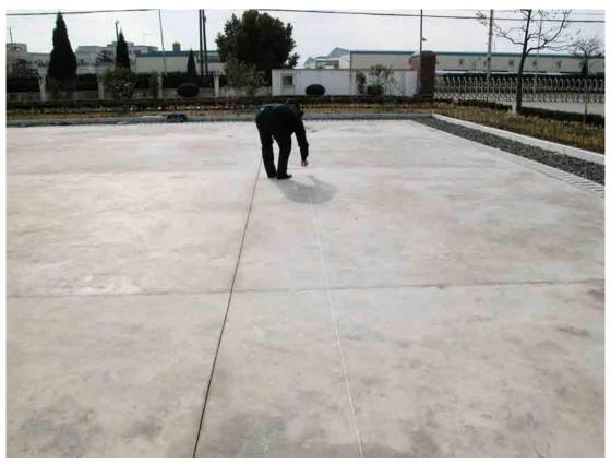
First step: Based on the basketball court to identify the location of all the white line and later snap the ink and carpenter's sink marker.
