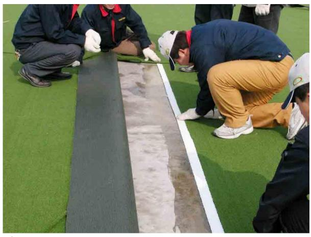
$16^{th}$  step: glue the joint between the white and green lawns (width is 15cm-20cm), clapped them together after air-dry.
