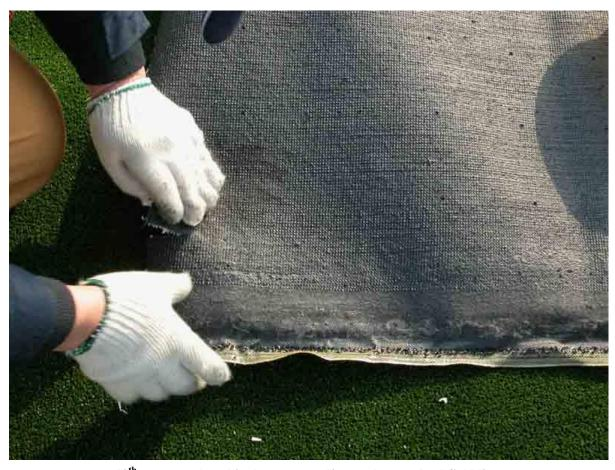
$12^{\text{th}}$  step: cut the white lawns according to the standard field line.
